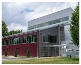
A new building envelope, pool upgrades, and field house HVAC system improved moisture and climate control in the multi-use space.
