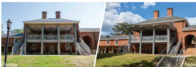
The lake side of the south pavilion was regraded to offer rear access to lower-level rooms, and the addition of a spacious deck improved access to Lake Chalgrove. The south pavilion now also boasts a large lounge and programming spaces on the first floor.
