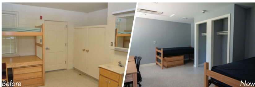
Interior improvements throughout all of Whitehouse included new flooring, walls, ceilings, and architectural trim. Sinks previously located in bedrooms were relocated to bathrooms enlarged by renovation of the arcades that link the pavilions, giving students more bedroom space and improved living quality.
