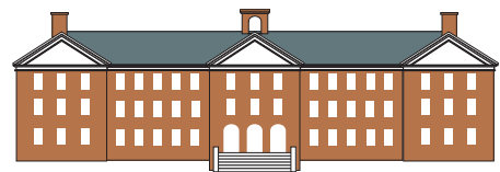
Kirby Fieldhouse: Ongoing multiphase project began summer 2021
